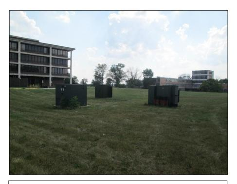
Photograph 33 – A view of pad-mounted electrical transformers.
